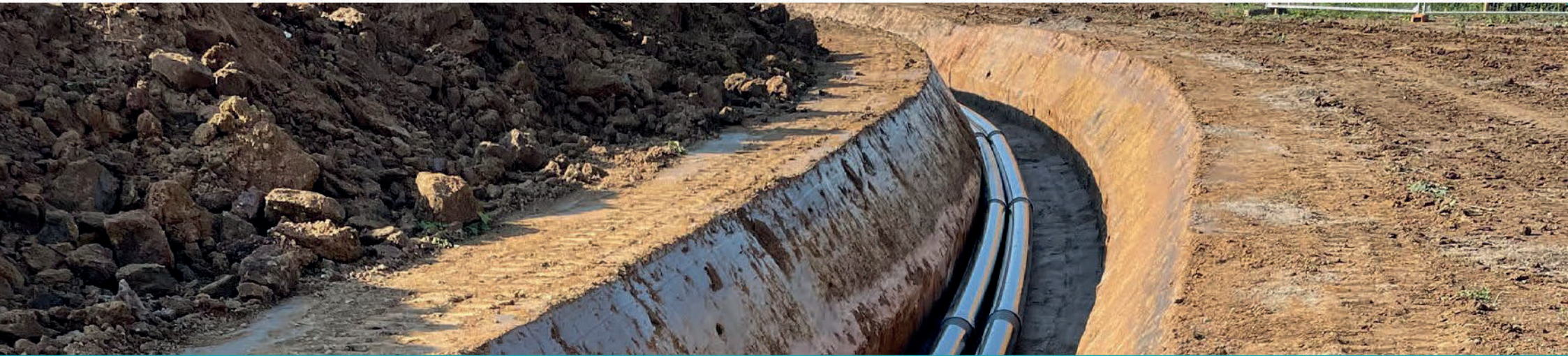
Open cut trench excavation and duct installation at Dogger Bank C HVDC cable route
